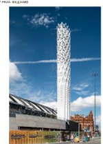
The final sections of Tonkin Liu's 40m-tall biomimetic 'Tower of Light' for
